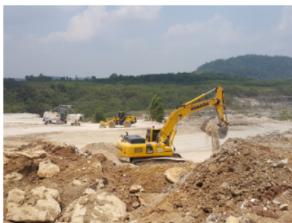
Figure 4. Stripping Cover Ground Layer Using 30 T Excavator
