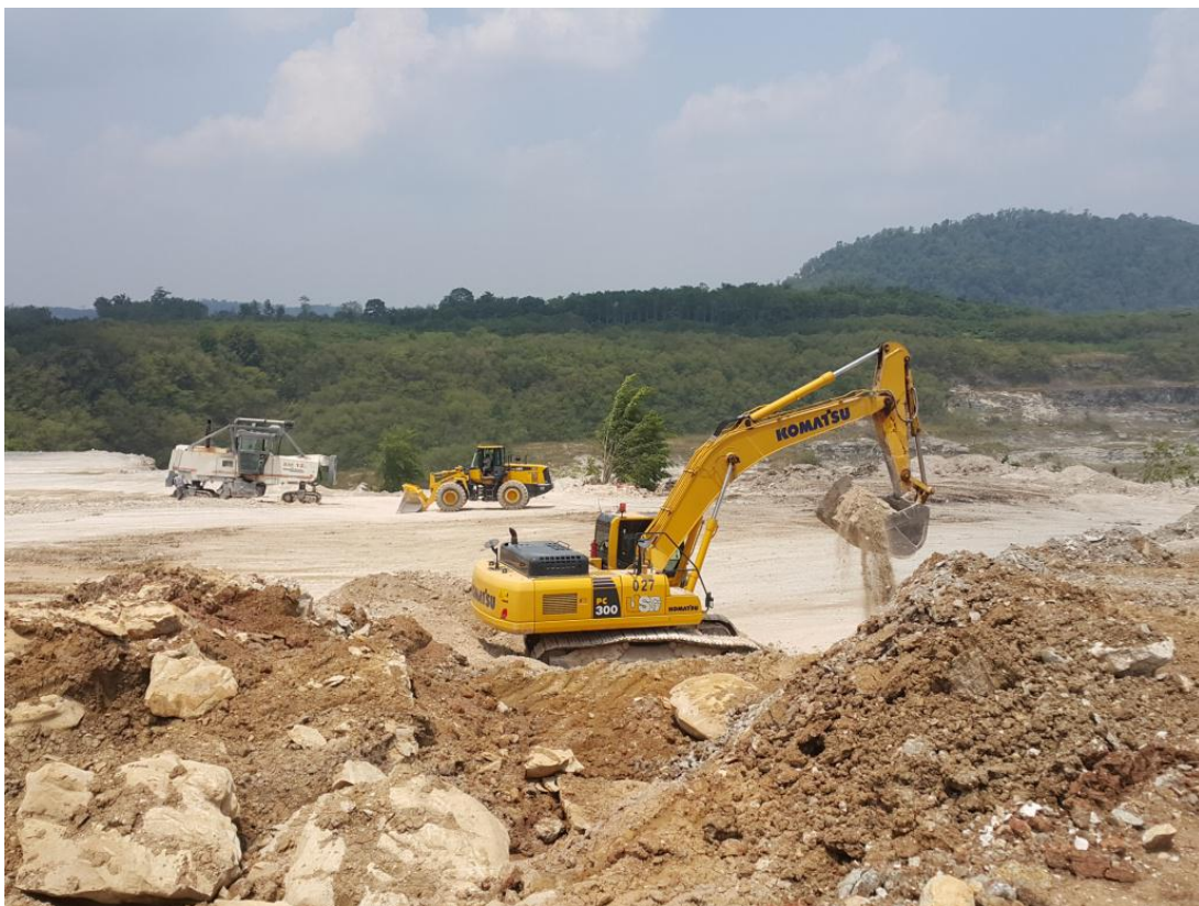
Figure 4. Stripping Cover Ground Layer Using 30 T Excavator
