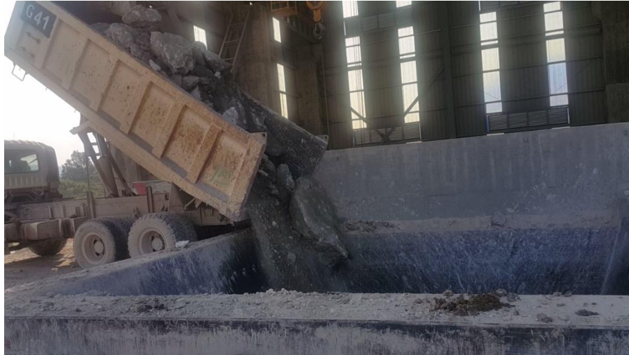
Figure 7. Dumping Activities at the Crushing Plant.
