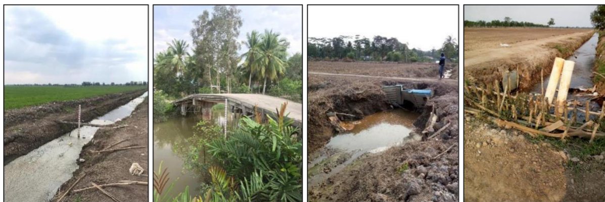
120 Figure 1 Tidal lowland canals condition in Muara Telang Sub District
