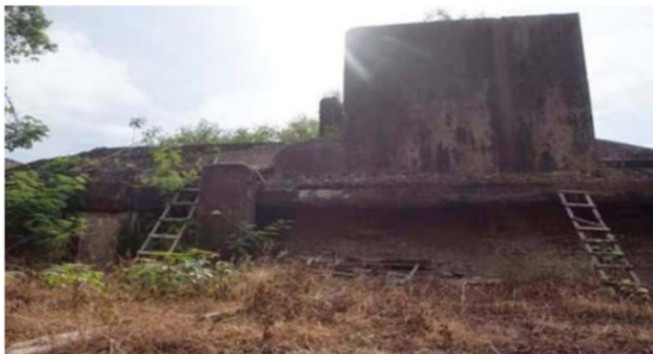
Gambar 3.8 Bunker Charitas Tampak Samping
