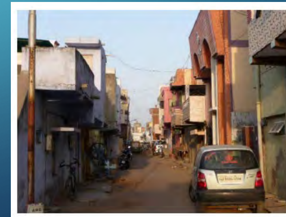
Figure 2. Buildings with off-set infill walls line this street.
