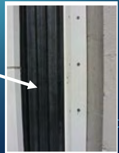
Figure 5. A close-up of the flashing covering the seismic gap.
