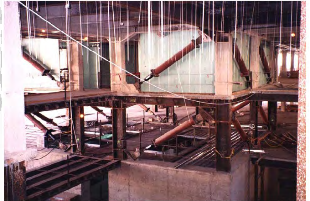
FIGURE 30 SAN FRANCISCO CIVIC CENTER DAMPER INSTALLATION
