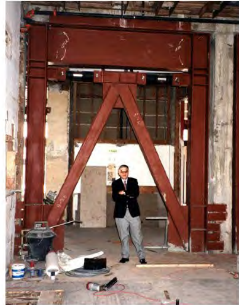
FIGURE 33 HOTEL WOODLAND - INSTALLATION OF DAMPERS
