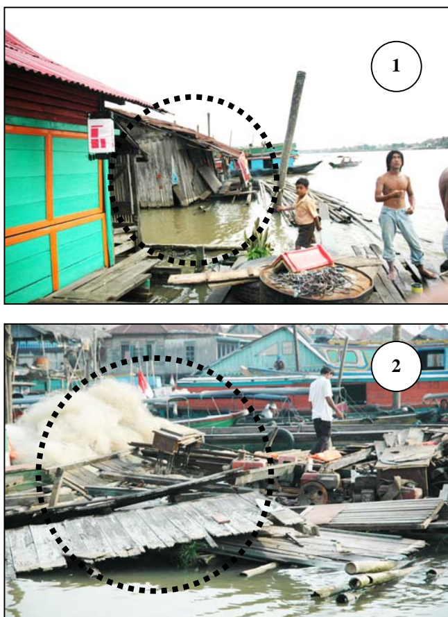
Figure 1. Raft house damaged (picture no.1) and then collapsed (picture no.2). Source : Field survey, 2006
