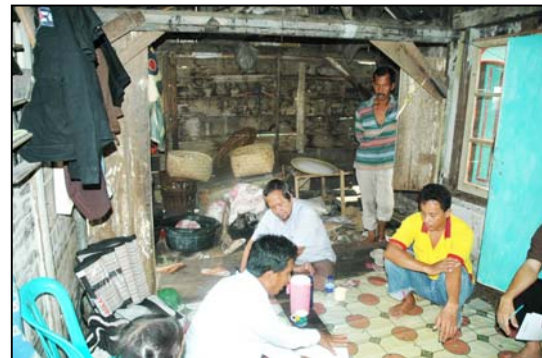
Figure 7. Inventory process raft houses damaged by Fitra NGOs, Provincial Public Works Department and community leaders. Source : Field survey, 2006
