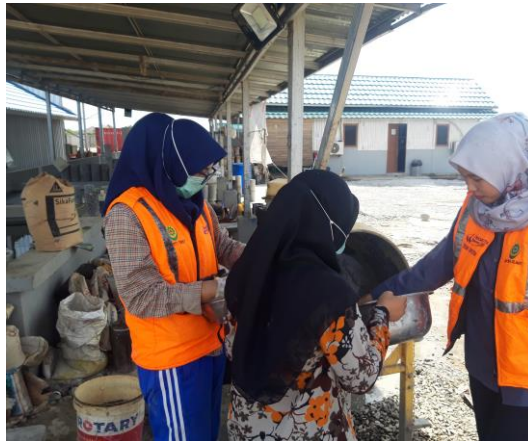
Gambar 3.20. Proses Pengecoran Pervious Concrete
