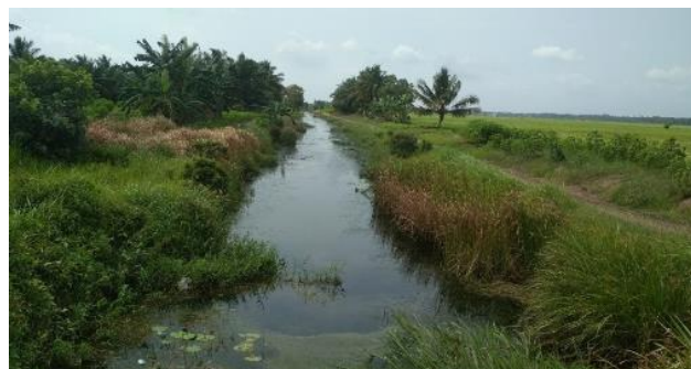
Figure 4. Condition of Secondary P17-6S Channel in 2019
