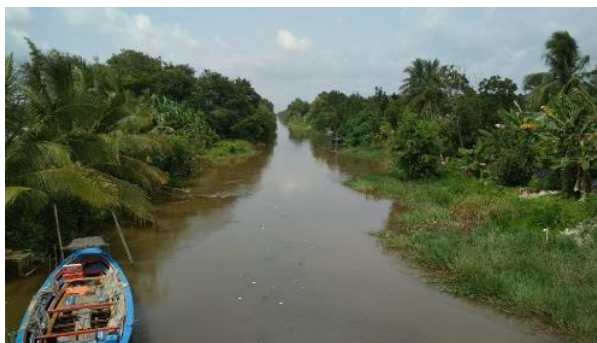
Figure 3. Condition of Primary 17 Channel at Telang II in 2019
