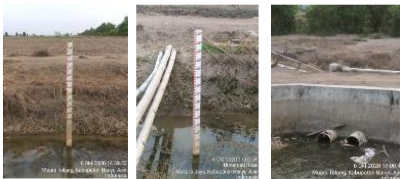
Figure 9. Condition of water control gate operation and initial growth of rice crop in land at 6 October 2020.
