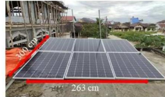
Fig. 10. The cross-sectional area of the panel
