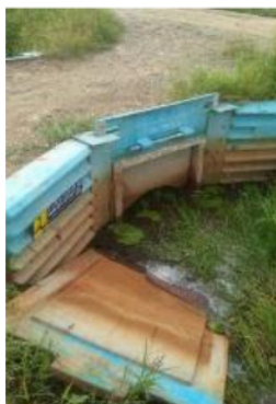
Figure 9. Watergate is opened to put high tidal water when crops is entering generative phase (March 2019)
