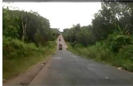
Figure 5. Peninggalan – Sei Lilin National Street (KM 135)
