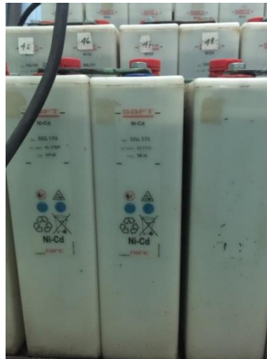
Gambar 3.5 Name Plate Sel Baterai Saft SNL 170.
