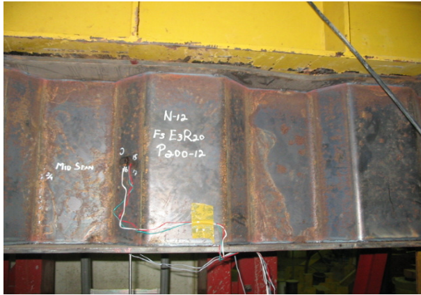
Figure 12 Local buckling of the top flange of specimen N12.
