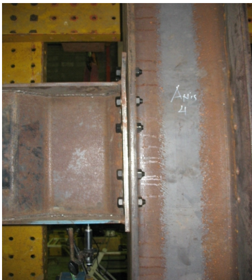
Figure 13 Small deformation of extended end-plate connection in “Y-shape” manner.
