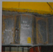
Figure 7: Failure mode of beam on sub-assembly tests
