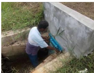
Figure 8. Tertiary gate installed at outside (tide water can not enter) with water management objective is maximum drainage.
