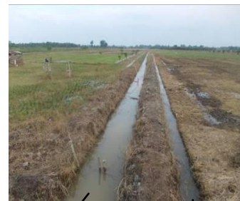
Tertiary channel collector channel
