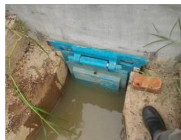
Figure 8. Tertiary gate installed at outside (tide water can not enter) with water management objective is maximum drainage.
