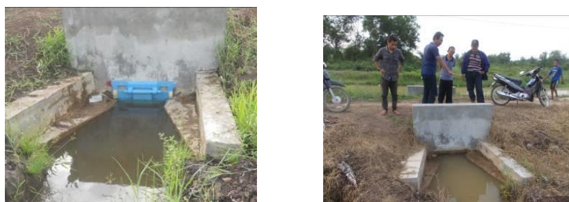
Figure 5. Operation of tertiary water gate as supply (holding water during low tide period)
