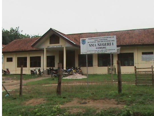
Figure 1. School Building of SMA Negeri 1 Cengal
