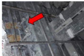
(b) IJT-03 shear connector
