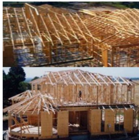
Fig. 4. Pre-fabricated timber frame system
