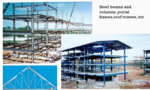
Fig. 3. Steel framing systems
