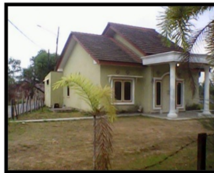
Fig. 2a. Permanent House/high income
