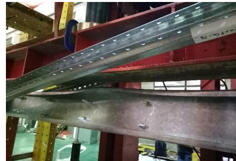
Fig. 17. Beam flange have crushed
