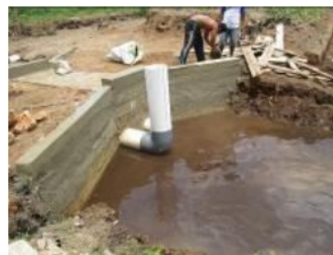
Figure 9. Operation of goose neck-type water gate to retain water
