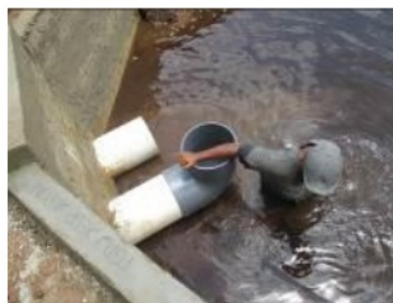
Figure 9. Operation of goose neck-type water gate to retain water
