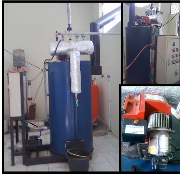
FIG. 1. The fire tube boiler.
