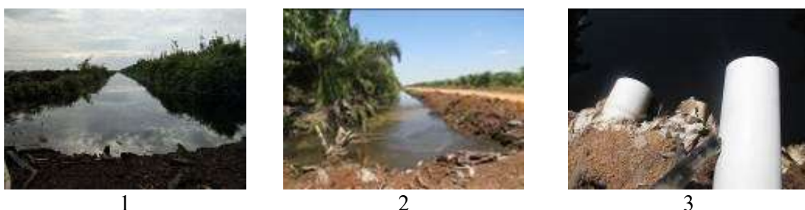
Figure 6. The multi-store block technique (photos 1 and 2: [12]); (3) the secondary channel blocking in an oil palm plantation and control overflow.
