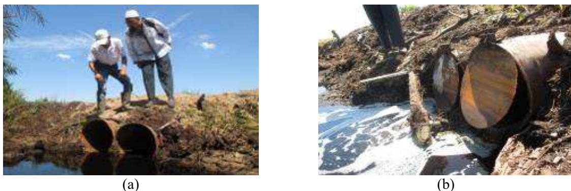
Figure 3. The main drainage systems including valve door; (a) the inside; (b) the outer lead toward to free waters or disposed region (swamp).
