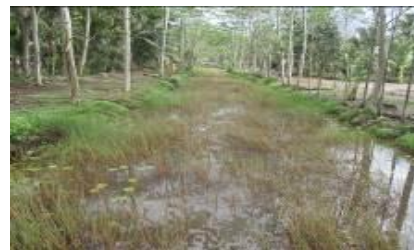
Figure 5. Condition which need to be rehabilitated
