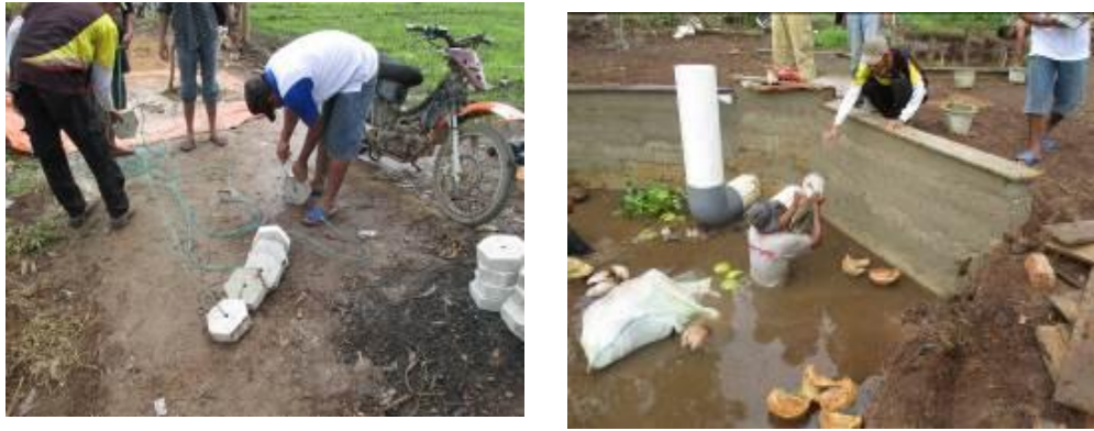
Figure 14. Application of smart conblock in channel
