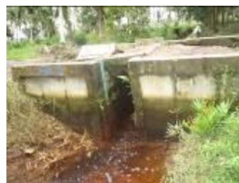
Figure 4. Valve-type gate at tertiary channel which is wide but too small to resist vehicles load.
