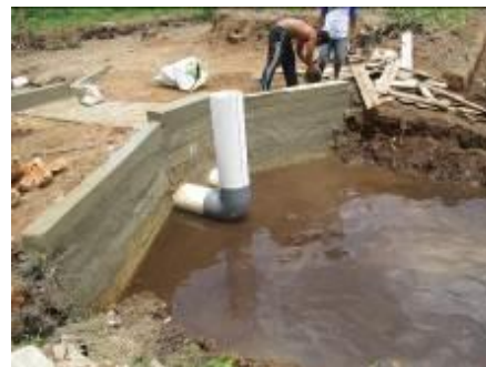
Figur 9. Operation of goose neck-type water gate to retain water
