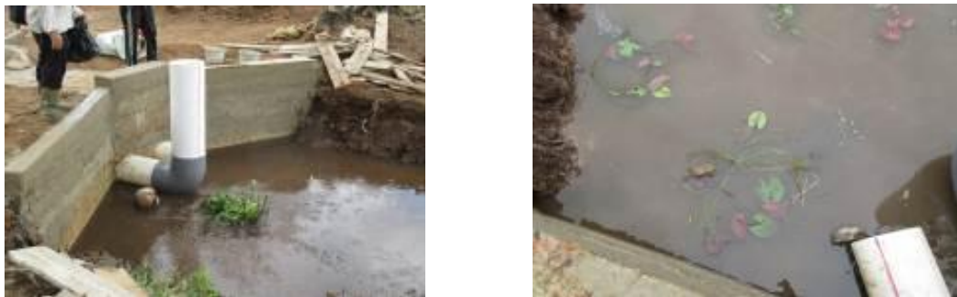
Figure 15. Application of phytoremediation using water hyacinth and lotus in channel
