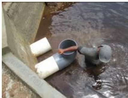
Figur 9. Operation of goose neck-type water gate to retain water
