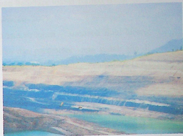
b. Lereng Keseluruhan ( Overall Slope )
