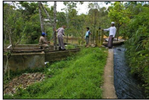
Gambar 8. Saluran lebar 90 cm kedalaman 45 cm Debit = 0.282 \text{ m}^3/\text{detik}
