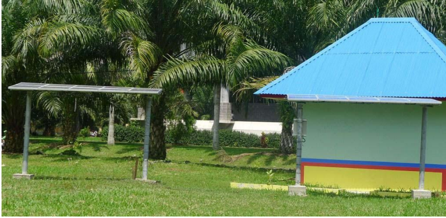
Figure 6 PV Facility at Sriwijaya University, Indonesia
