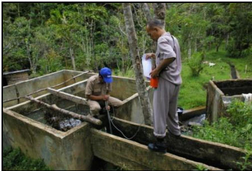
Gambar 9. Inlet Mikro hidro lebar 45 cm kedalaman 45 cm Debit = 0.125 \text{ m}^3/\text{detik}
