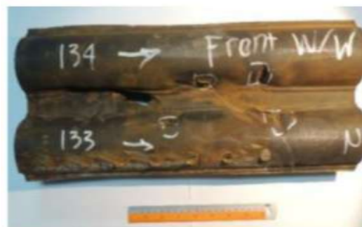
Figure 3. Waterwall Tube Boiler
