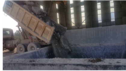
Figure 7. Dumping Activities at the Crushing Plant
