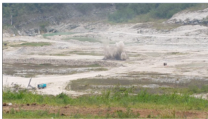
Figure 5. Blasting Activity PT. Semen Baturaja (Persero) Tbk
