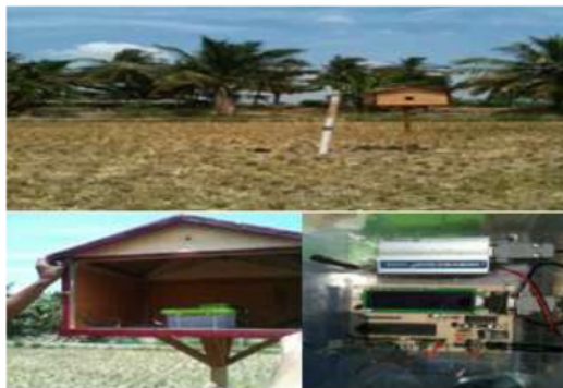
Figure 7: Sensor Equipment Water level
