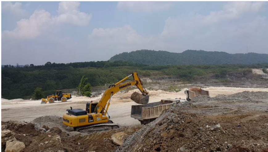
Figure6. Activities of Loading Materials into the Dump Trucks.
