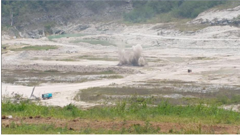
Figure 5. Blasting Activity PT. Semen Baturaja (Persero) Tbk.
