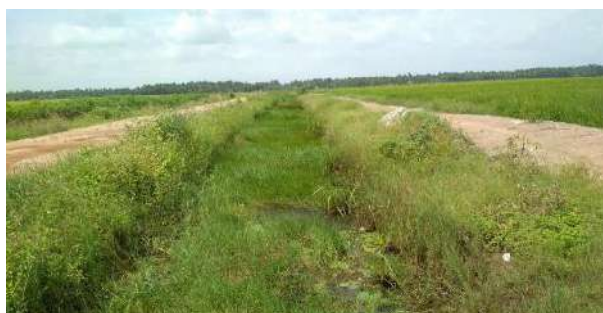
Figure 5. Condition of Tertiary Channel at TC 7 P17-6S in January 2019
