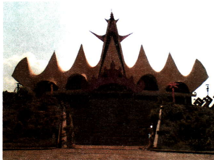
Picture 13: SIGER TOWER, the Pride of Lampung Province
