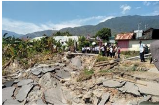
Figure 1. The condition of the liquefaction disaster that occurred in the Petobo area
