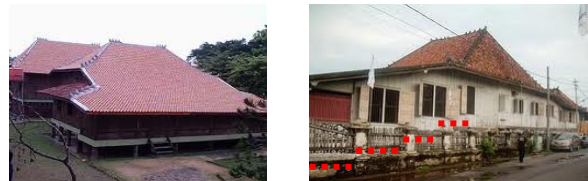
Figure 2: (left) The Roof Form Limas House, and (right) Split Level At Limas Main Room Source: (left) www.scycrapercity.com ; (right) www.rumahlimasPalembang.blogspot.com
