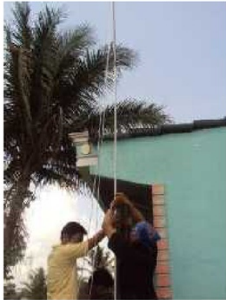
Figure 4: The head of pump is raised by enlengthened the supporting pipe.
