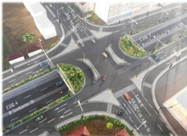
Fig. (2). Underpass construction at Patal-Pusri intersection.
