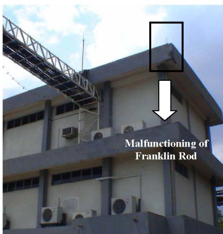
Fig. 1: A building structure equipped with standard rod at central and extreme edge of the building still being damaged by lightning stroke.
