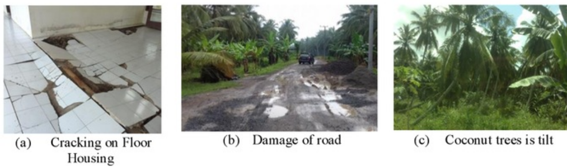
Fig. 4. Direct Impact of Land Subsidence.
