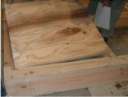
Figure 6. Sheathing floor beams with sugi plywood
