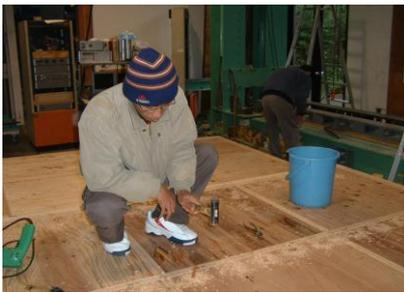
Figure 8. Nailing sugi dowels to panels
