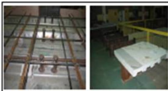
Figure 3. Installation of Studs, metal decking, and composite
