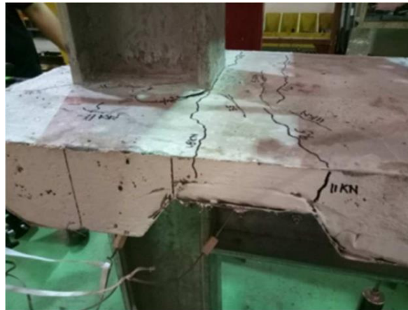
Figure 8. Transverse cracks on concrete slab
