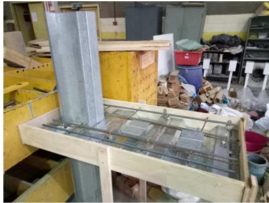
Figure 5. Reinforcement bars and BRC inside the slab deck for Specimen 1
