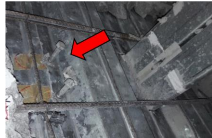
(b) IJT-03 shear connector
