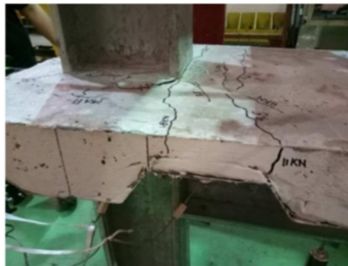
Figure 8. Transverse cracks on concrete slab
