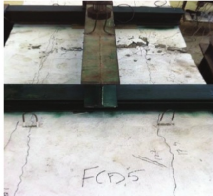
FIGURE 7. Longitudinal crack, CFS thickness 3mm
