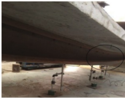
FIGURE 6. Buckling of steel beam flange, CFS thickness 2mm
