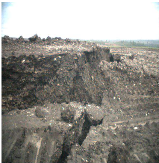
a. Tension crack at the crest of failure
