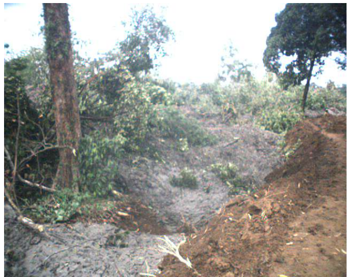
b. One view at the toe of the failure
