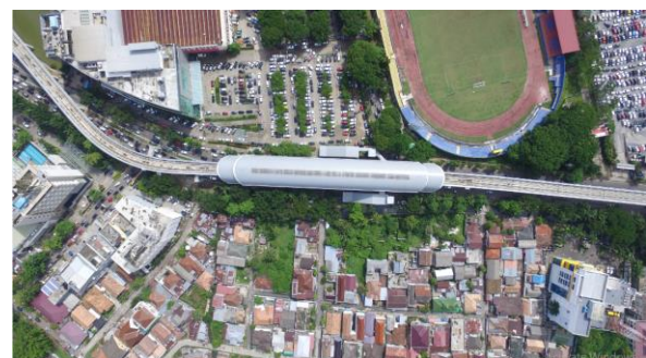
Figure 4. TOD area Bumi Sriwijaya LRT station
