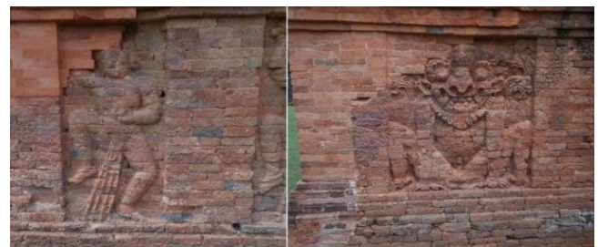
Fig. 8 The use of new bricks on the wall that have reliefs
