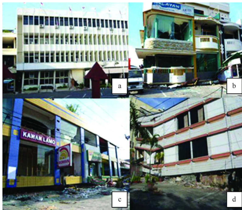
FIGURE 2. The Padang earthquake on September 30 & October 1, 2007: a). The Office of DPU Padang experienced a soft story on the 1 st floor but it was still survived, b). The shophouse 3 stories experienced severe a soft story at the 1 st floor. This floor collapsed, and the 2 nd & 3 rd floors fell on it, c). & d). The commercial building experiencing a severe soft story at the 1 st floor. This floor collapsed, and the 2 nd & 3 rd floors fell on it (source: http://www.perencanaanstruktur.com/2010/10/bentuk-keruntuhan-bangunan-saat-gempa.html ).
