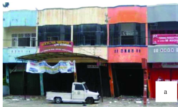
FIGURE 8. Weak story due to reversed pyramid form can be minimized by using flexible and light materials like aluminum composite
