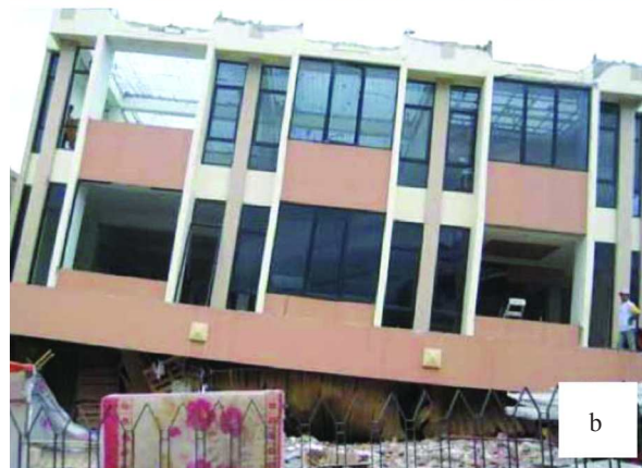
FIGURE 9. West Sumatra Earthquake in 2009, a). Ruko/ shophouses undergoing residual drift, b). The first floor of the shophouses collapsed (source: Wilkinson et al. 2012).
