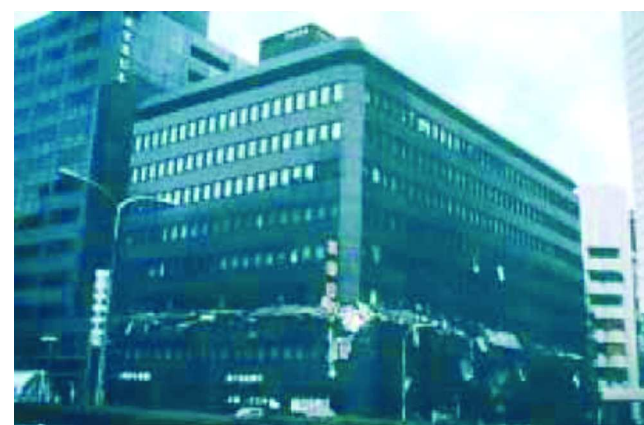
FIGURE 4. The Kobe Earthquake of 1995, the third story of the commercial building was lost and the above stories fell on it (source: Bachmann 2003).
