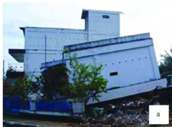
FIGURE 9. West Sumatra Earthquake in 2009, a). Ruko/ shophouses undergoing residual drift, b). The first floor of the shophouses collapsed (source: Wilkinson et al. 2012).
